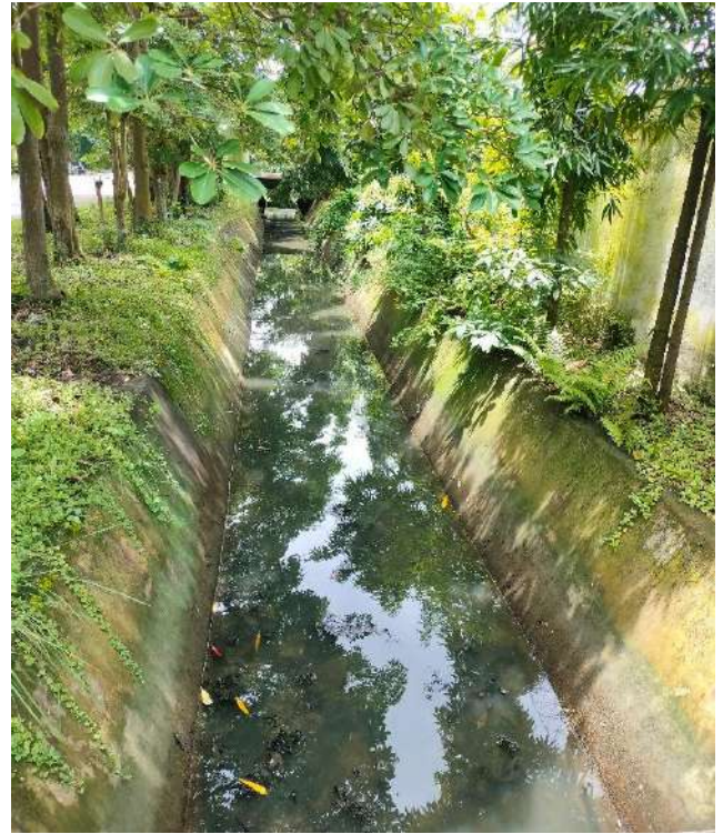
Plate No: 4 Open Drainage System
